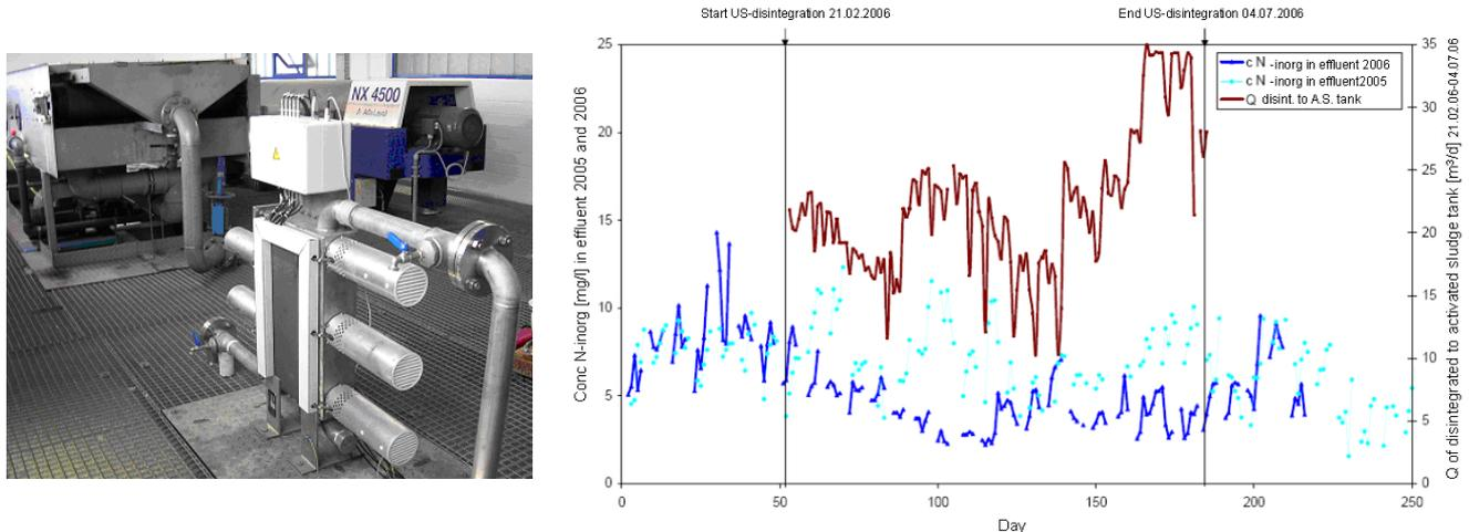
Figure 4: Installation at Bünde WWTP and results. The lower N-inorganic concentration in the effluent of Bünde WWTP during the sonication period in 2006 corresponds to a higher degree of efficiency with regard to denitrification.
